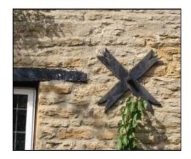
The house preceding number 21 is Forge Cottage, which is of a similar age – note the tie plates in wall. They are there to stop the walls bowing out.
